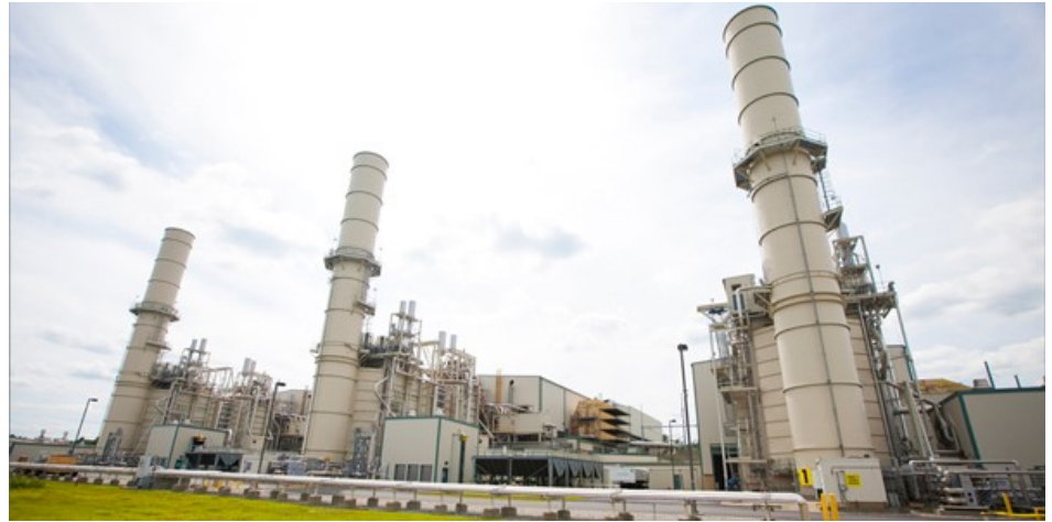
Dynegy's 827-MW Lake Road combined cycle plant, Dayville, Conn. | Alstom
