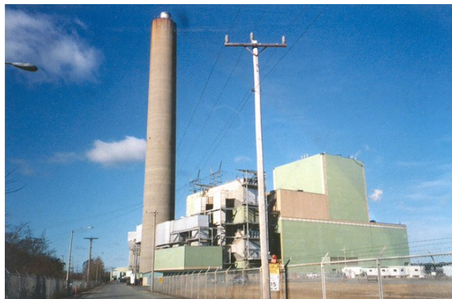
Canal Generating Station | EPA
