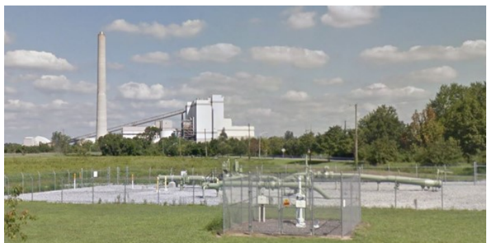
Ares' 242-MW power plant in Logan Township, N.J. | © RTO Insider
